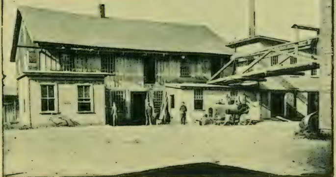
LYON'S Iron Works and Foundry
